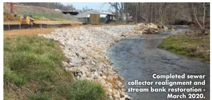
Completed sewer collector realignment and stream bank restoration - March 2020.
